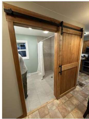
Bathroom Door Widening
