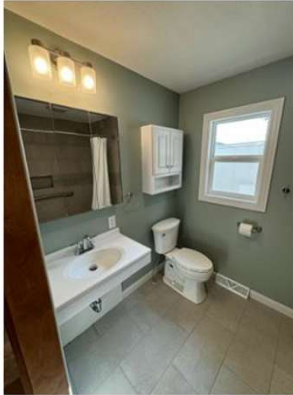
Wall Hung Vanity Relocation of the Toilet
